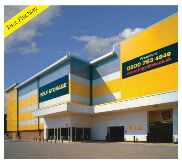
Big Yellow Self Storage East Finchley is constructed from materials with a high recycled content including: steel; aluminium window frames; particle board flooring and walls; breeze blocks and solid insulation.
