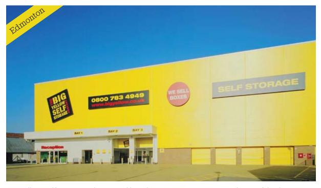
Big Yellow Self Storage Edmonton, like other more recent stores in the portfolio, has energy efficient cladding with solid insulation that reduces daily and seasonal temperature variations within the storage area. No heating and cooling is required in about 97% of the store area.
